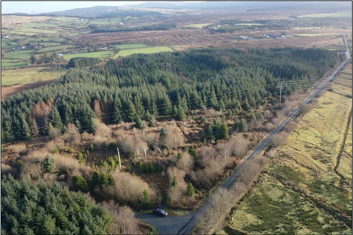
Plate 3: View of proposed area for battery storage southeast of current sub-station, facing northeast
