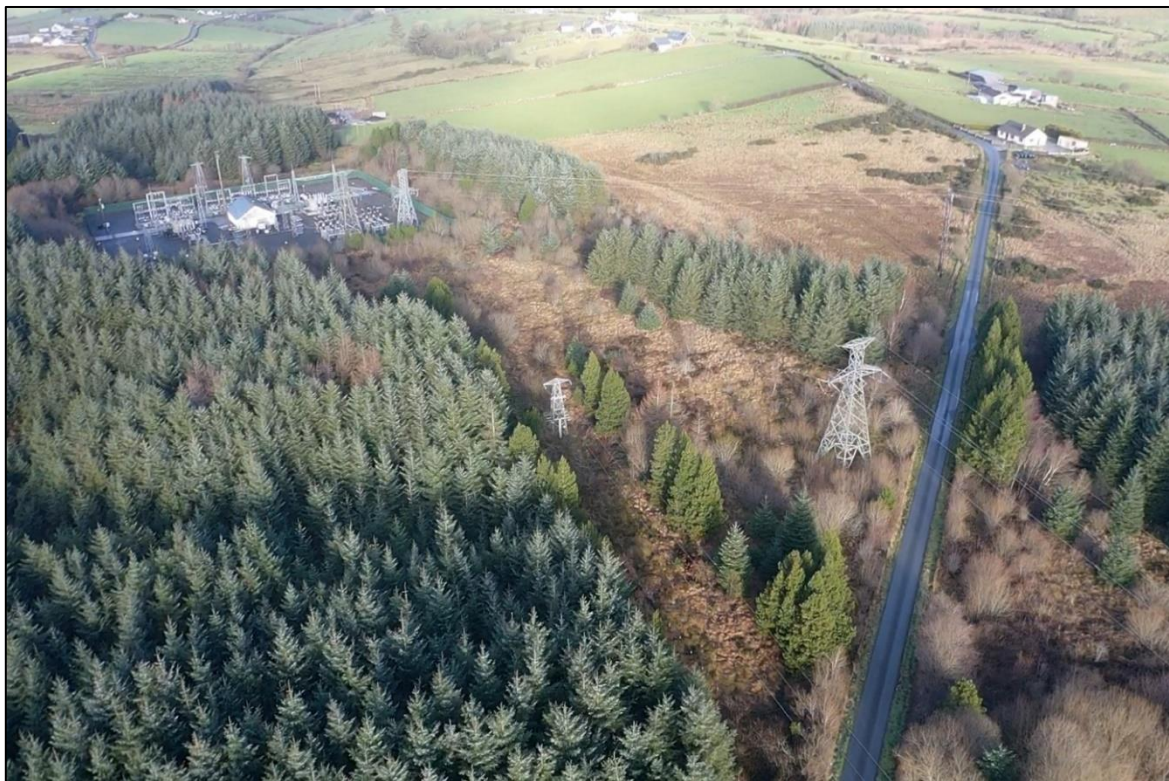
Plate 2: View of location of test pits 1 and 2 (under powerlines) southeast of current sub-station, facing northwest
